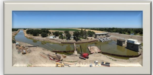
Karnak Pump Station
